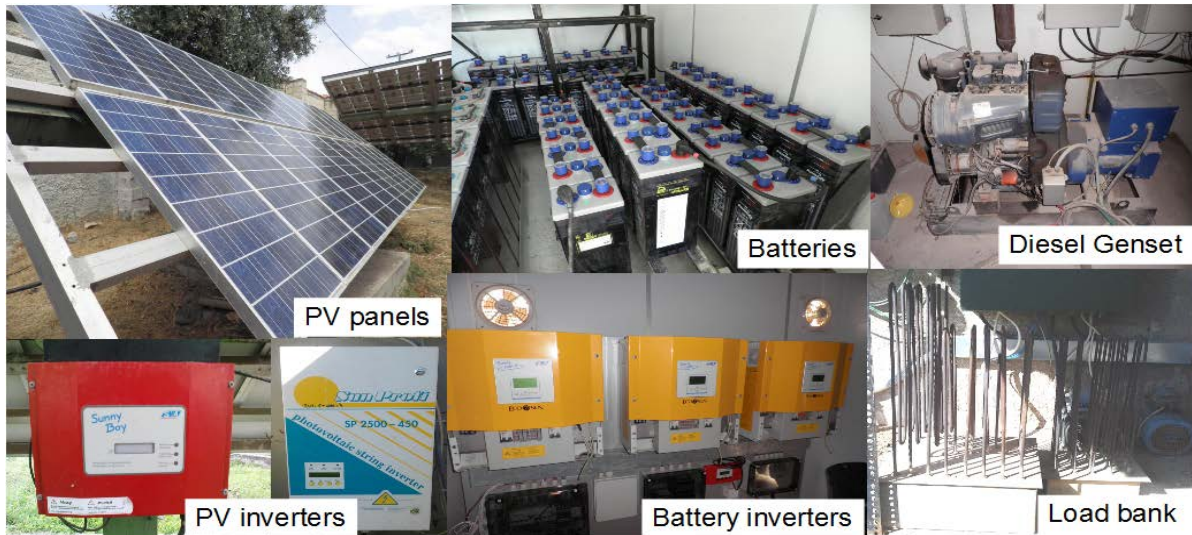
Overview of microgrid's main components
