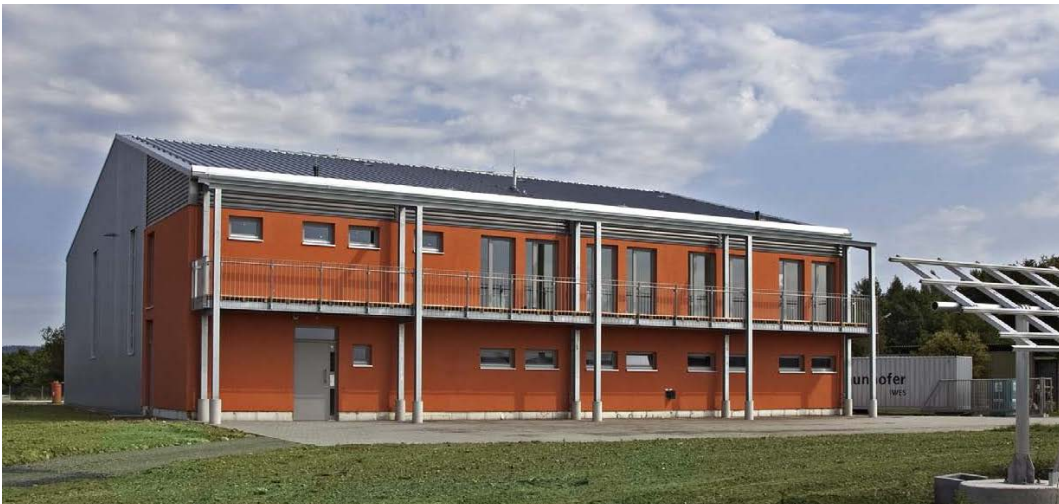
Figure 1: The main building of IWES-SysTec with the labs SysTec PNI and SysTec TPE
