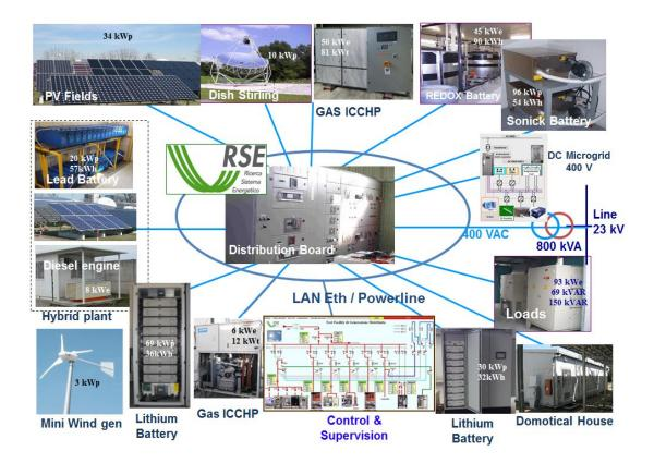
A Supervision and Control system has been developed in order to monitor and control all installed resources.
